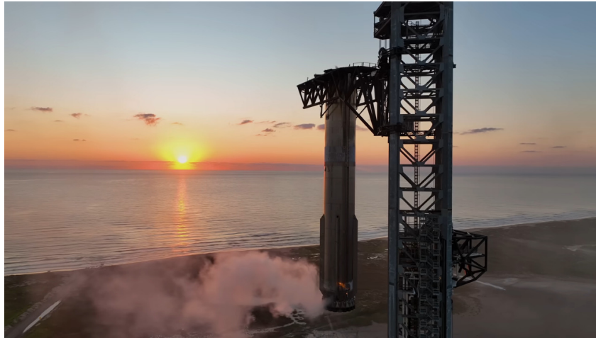
Figure 16: The booster empties its tanks after being caught
